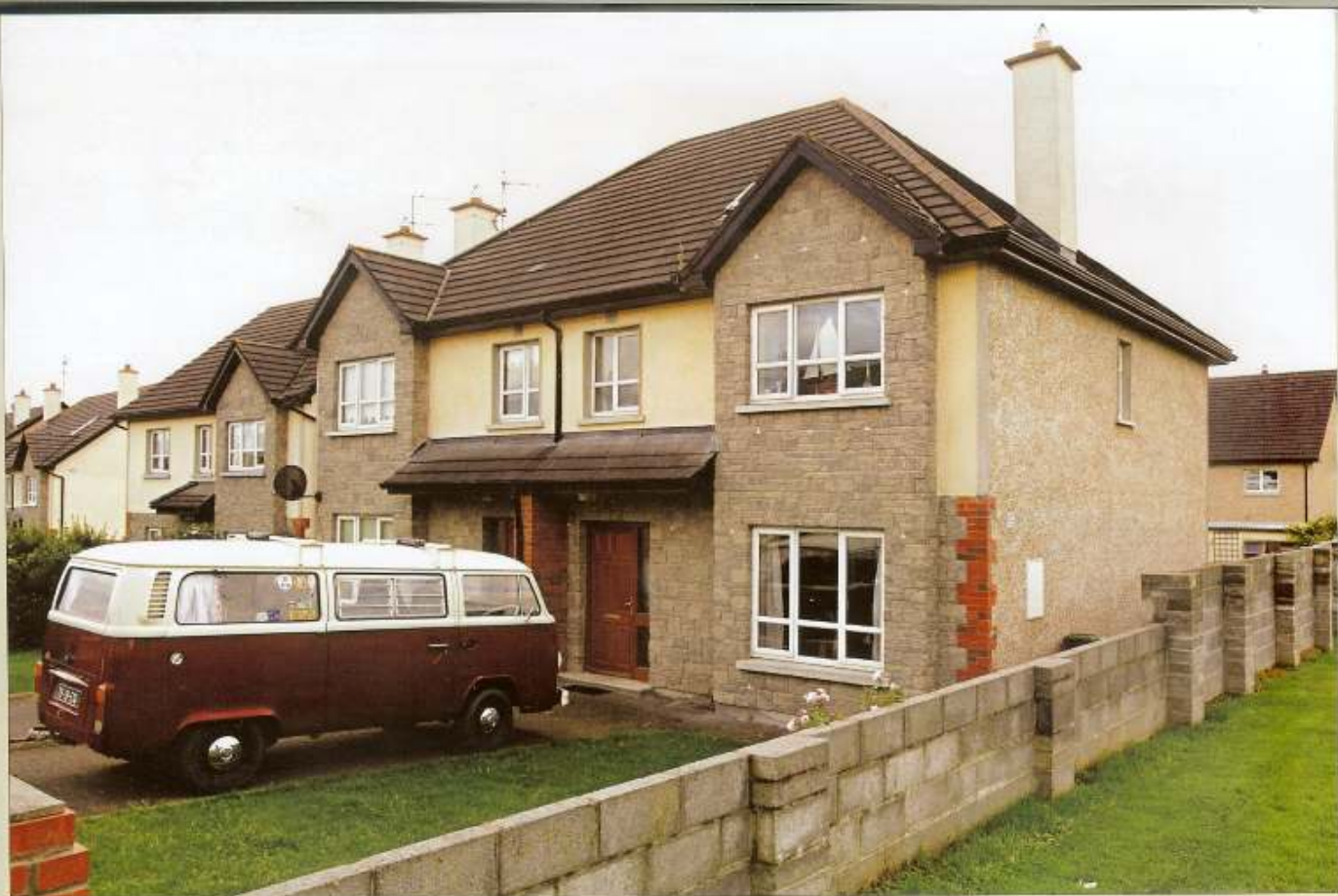
(above) Energy consultant Paul Kenny upgraded his semi-detached home in August and already is noticing the difference, using rooms now that were too cold before; (below) motion and daylight sensors were installed beside light fixtures throughout the house
