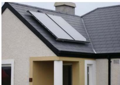
*4m<sup>2</sup> of solar panels on the roofs provide most of the resident's domestic hot water requirements*
